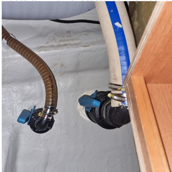
Waste tank valve located behind door under the sink
